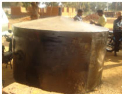
digester includes a masonry-lined cylindrical pit, metal guide-frame and gas-holder (dome) and two tanks (one each for input of dung-water slurry mixture and outflow of spent effluents, respectively). Construction is being monitored by our staff with adequate precautions.
